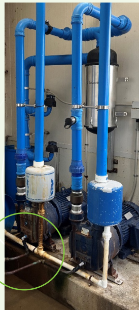
3 Example of a milk pump. There is no vacuum cylinder. It has standard diameter pipes.
