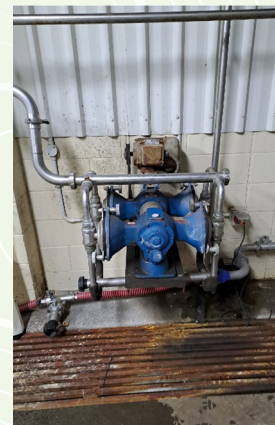
3 Example of a milk pump. There is no vacuum cylinder. It has standard diameter pipes.
